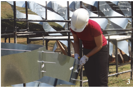
Figure 3. Pavilion being partially assembled.
