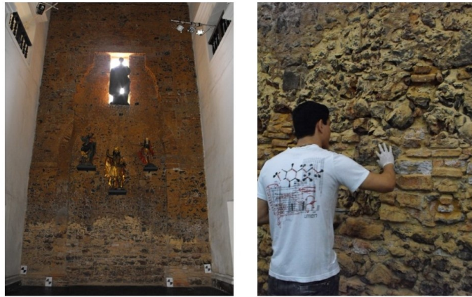
Fig. 2: Mixed masonry of stone and brick at Church of Santo Alexandre, in Belém, which presents salts crystallization problems in a level that compromises the conservation of (A) and sanitation mortar application for salt removal, as a result of the student Alexandre Maximo Loureiro master dissertation research, guided by Prof. Rômulo Angelica. C Santo Alexandre, Belém. Source: Thais Sanjad, 2011.
